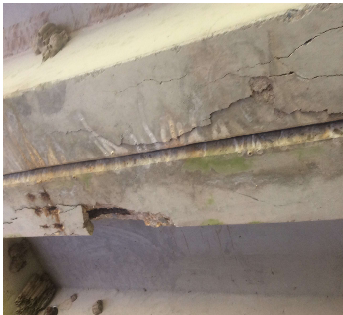
PHOTO 3 Description Span 3 units 3-4 have cracks, delams and spalls with exposed rebar to legs. Common units 5-7 this span.
