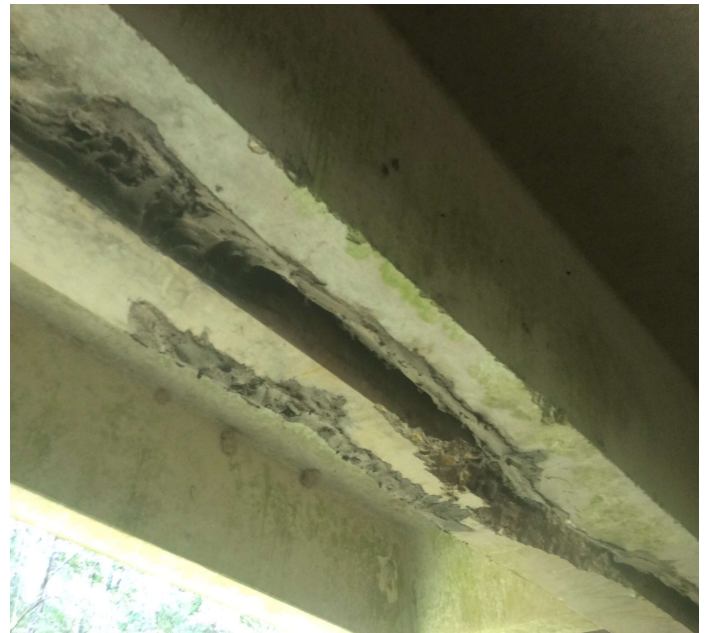
PHOTO 4 Description Span 1 units 7&8 have spalls with exposed rebar.
